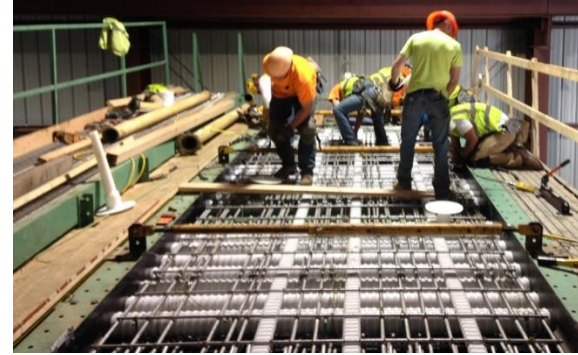
Stainless steel reinforcement costs 3-4 times as much as green epoxied and lasts at least 100 years
