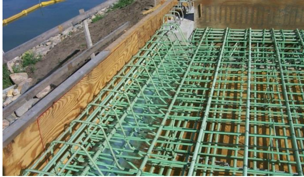
Standard green epoxied steel reinforcement lasts 50 years in our climate
