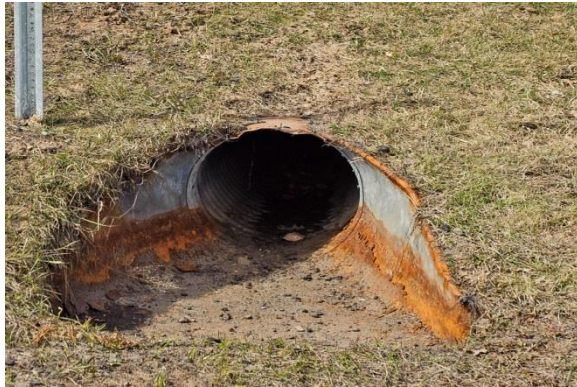
Standard 16 gauge galvanized pipe lasts 25 years
