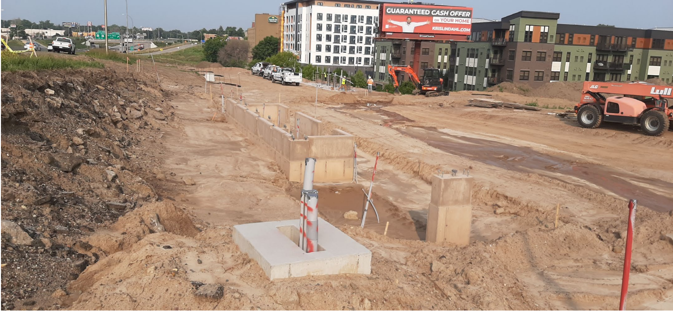
Hazel Station and Guideway grading
