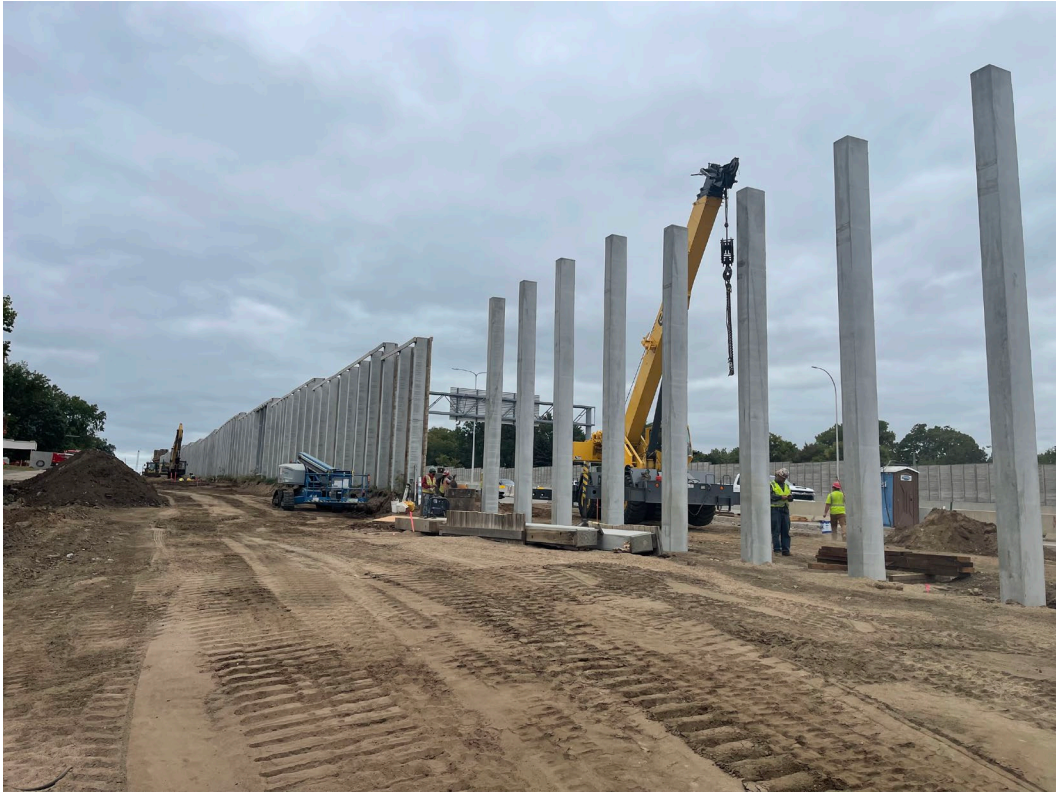
Hudson Road grading and Noise Walls
