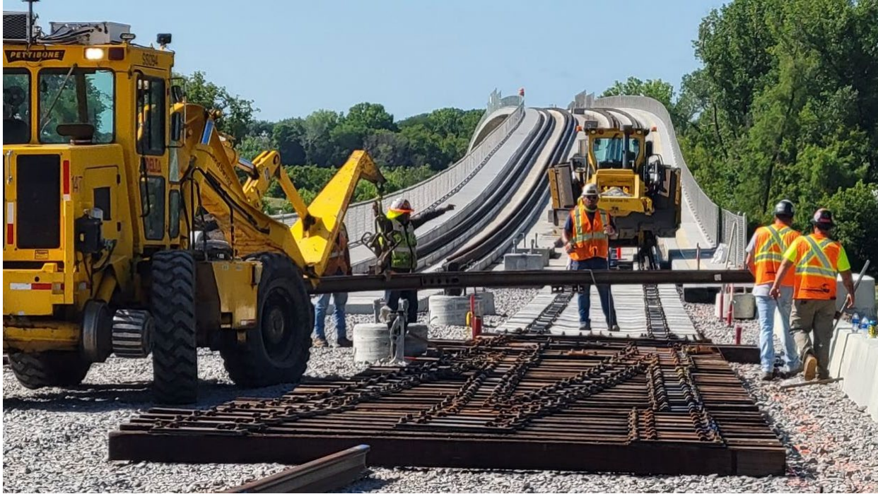
Special Trackwork at Minnetonka-Hopkins LRT Bridge
